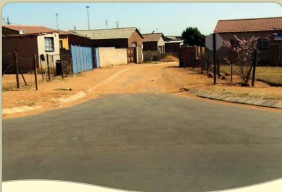
Yes, the roads are being upgraded and tarred
